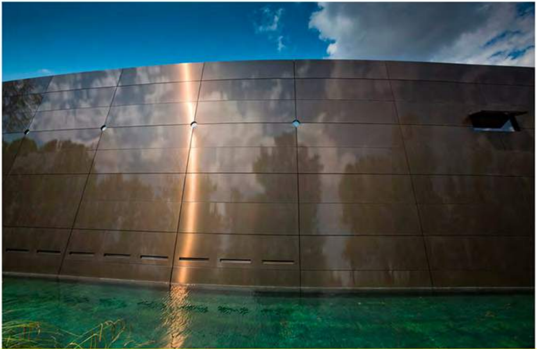
the structure is made of concrete, metal and glass
